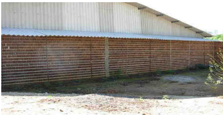
Figure 2 Porous wall (inlet)
